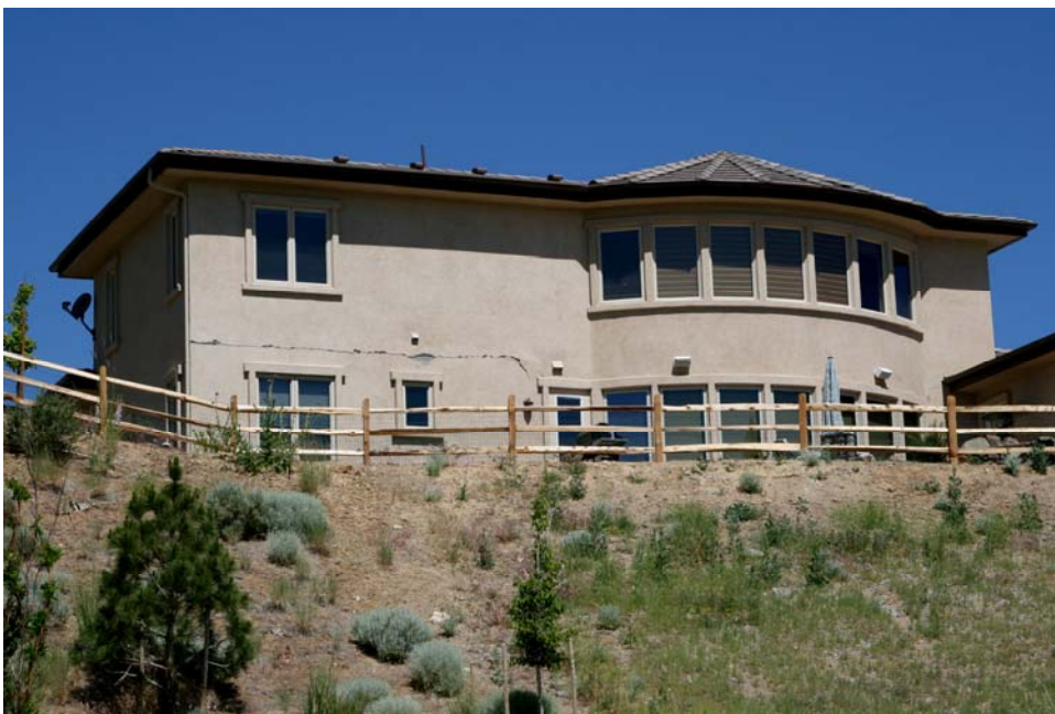
Figure 19 Overview of house shown in figure 18. Crack is on the left side of the building between the first and second stories.
