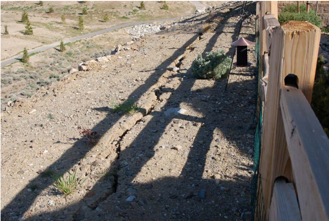
Figure 28 shaking and settlement fracture along the upper part of a large, three-tiered rockery wall. Total settlement was about 7 inches (17 cm) in places.
