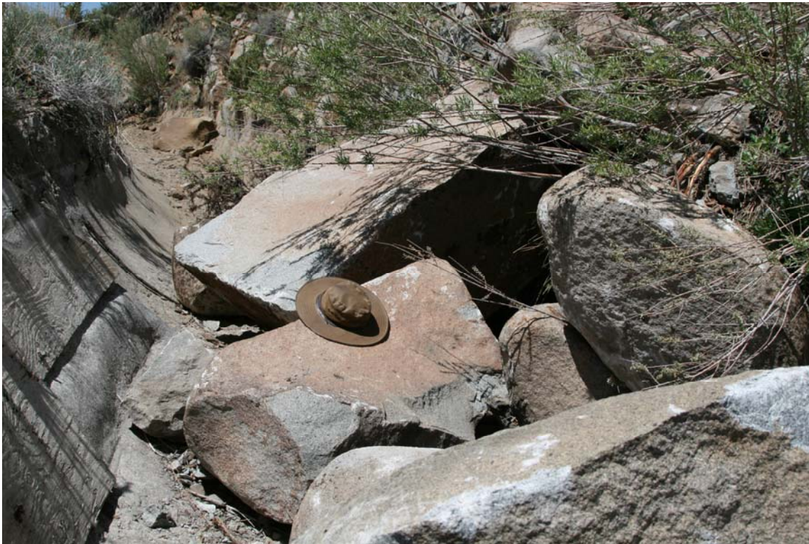
Figure 50 Rock slide of boulders that were coming down the hill and were trapped by the water canal.
