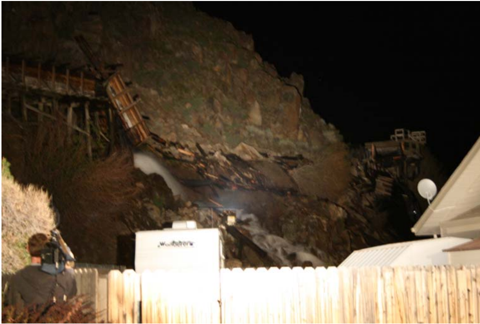
Figure 10 A rock fall broke the water flume and caused water to flow near houses.
