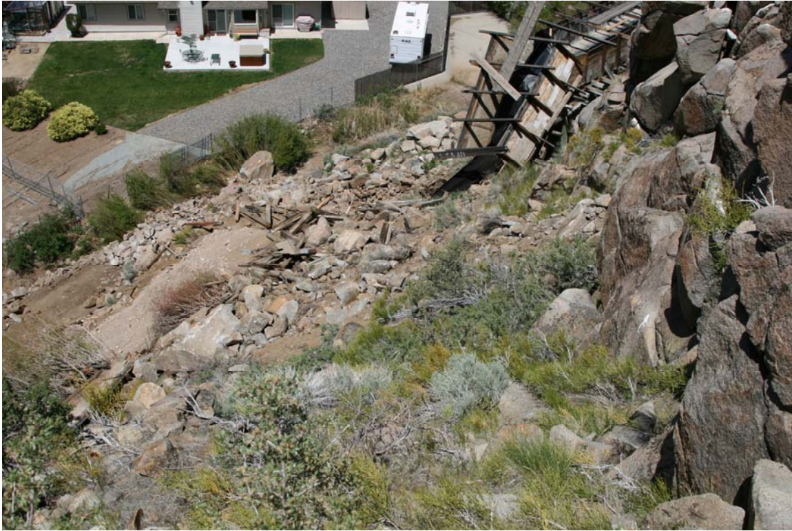
Figure 46 Part of the rock fall that damaged water flume.
